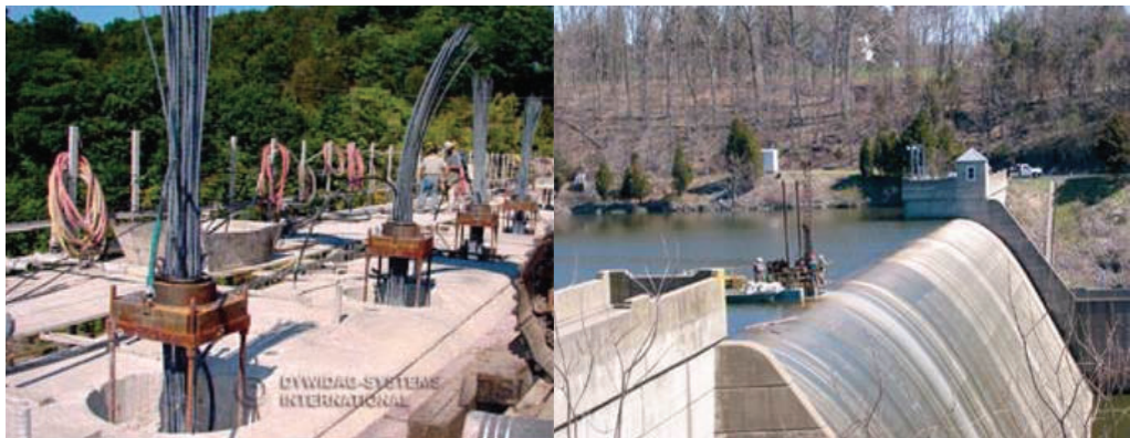
These two photos show the process of installing "rock anchors" on a dam as would occur if Alternative G – Stabilize-in-Place were implemented.
